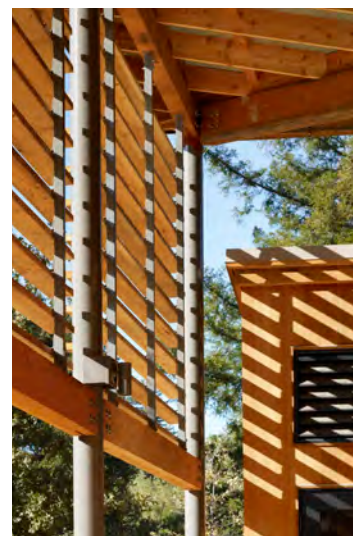
Wood sunscreens control solar heat gain and glare.
